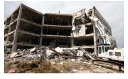
Brandenburg performed asbestos abatement, universal/special waste handling and disposal, and removal of PCB ballasts. Skid steer loaders were used on the interior upper floors to remove the debris within the structures. Elevator shafts were used as chutes and the waste was separated by commodity. Materials were either loaded as waste, stockpiled to be crushed or shipped to an appropriate recycling facility.
