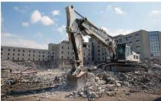
Brandenburg utilized its fleet of excavators to perform the structural demolition of the 700,000 square foot multistory buildings, ranging from one to six stories and an eight foot deep basement. Concrete slabs and foundations were removed and final site restoration was performed.
